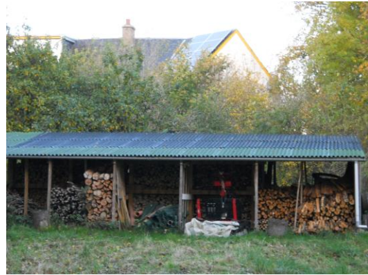
Log store and panels on the house
